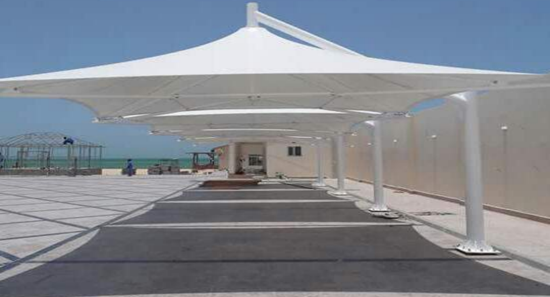
Car Parking Structure
