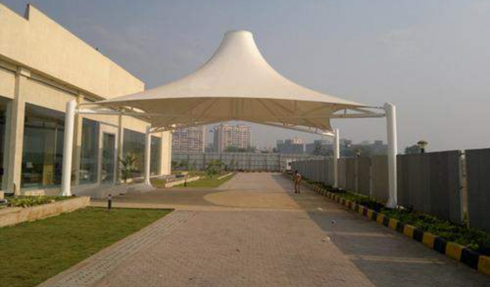
Cone Cover Structure at Resort in Mumbai
