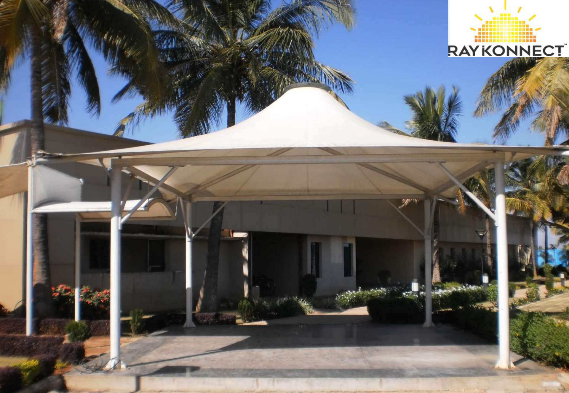
Cone Cover Structure in Bangalore
